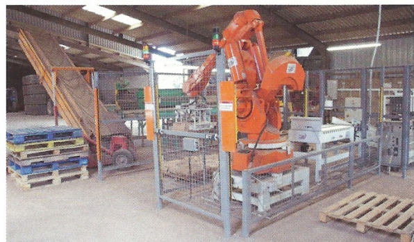
Twin cell robot palletizer installed at MS. Walker Shropshire
